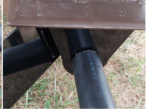
STEP 9 Slide pipe all the way onto end
