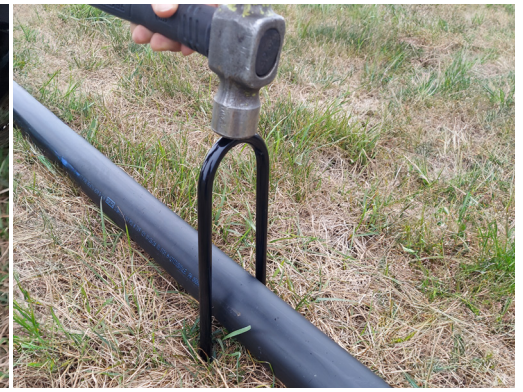
STEP 15 Straighten pipe and install U post halfway between hopper and front end of pipe
